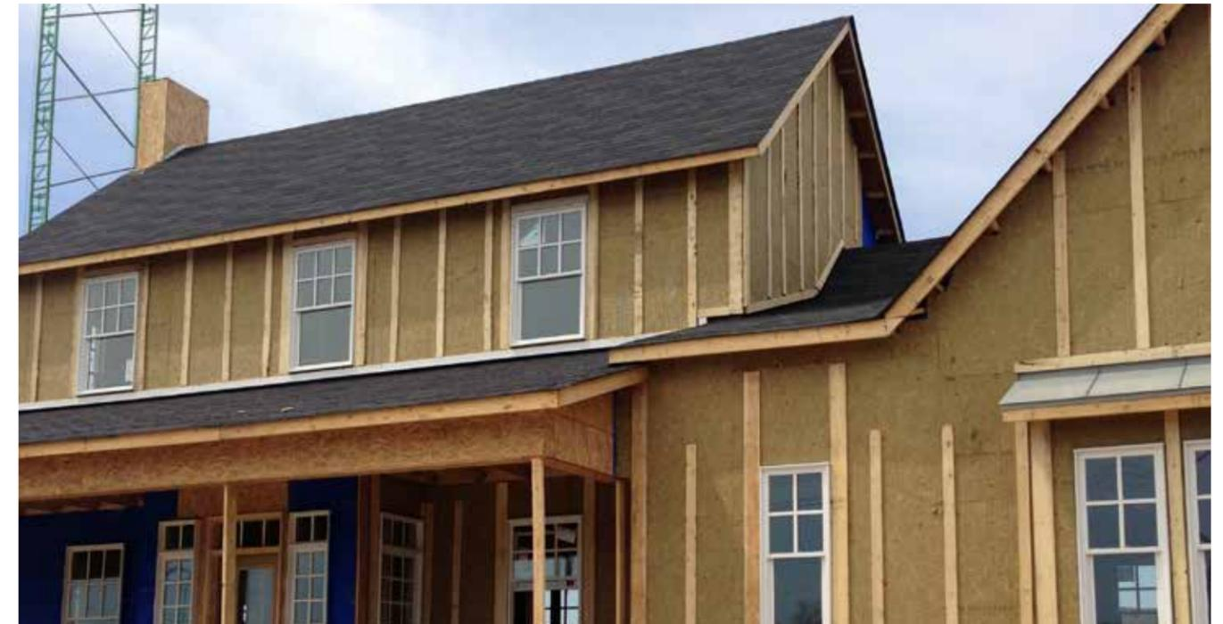
only risk to moisture damage is from an external leak. However, because the sheathing is kept warmer by the insulation, it is able to dry out faster, and in this wall
